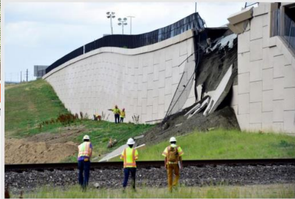
Land subsidence, side view of the collapse
